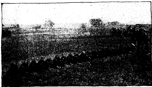
FIGURE 2.—Installed chemical projector battery.
