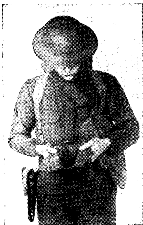
FIGURE 38.—INSPECT MASK. TWO. Examining facepiece.
